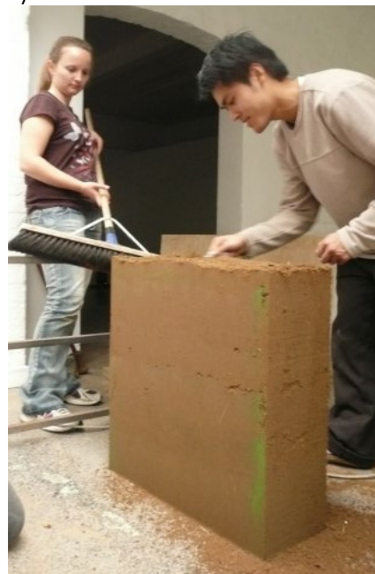
John tests the properties of a newly constructed section of a Whareuku wall.
